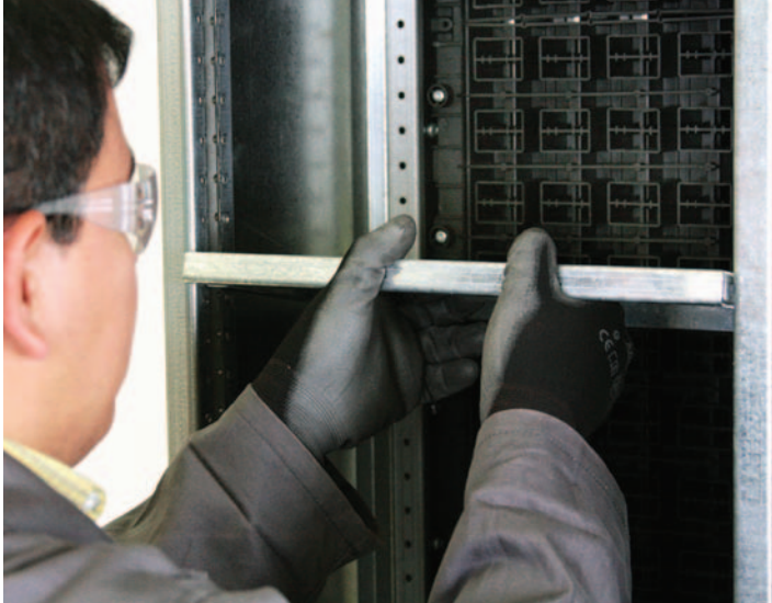
FIGURE 36. Dismantle Compartment Bottom Plates
