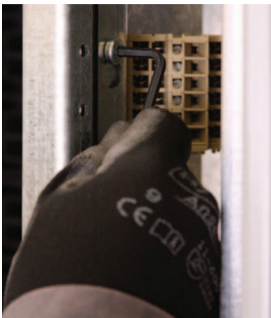
FIGURE 33. Uninstall the Control Terminal Block Support
