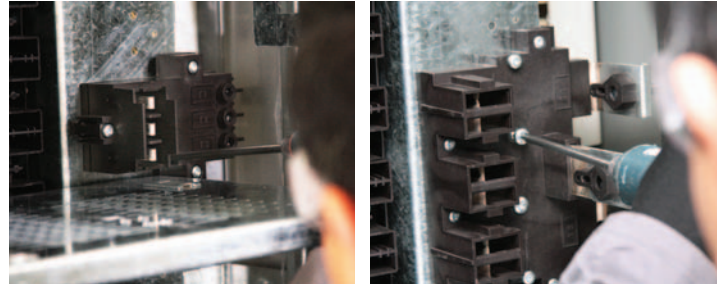
FIGURE 34. Uninstall Power Cable Connection
