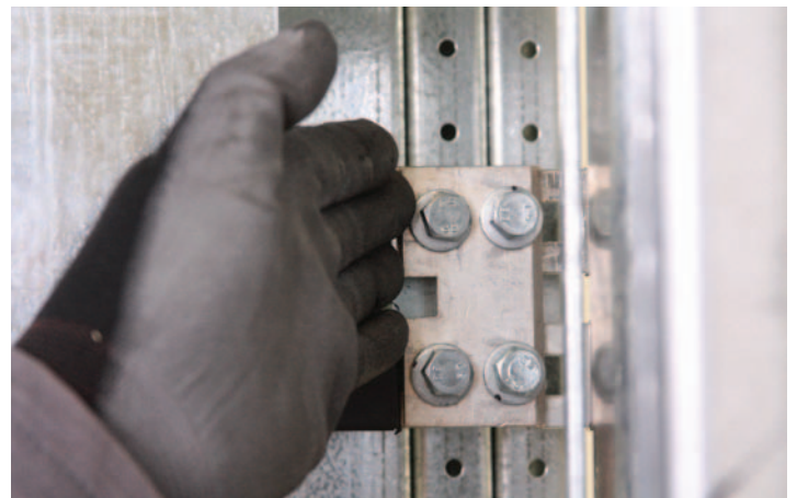
FIGURE 27. Slide the Link to the Adjacent Bus Bar
