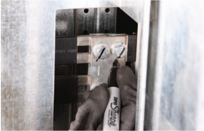
FIGURE 28. Frame Connection Using Spacer Bolts
